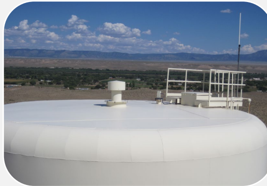
Batch Chlorinating Stored Water
