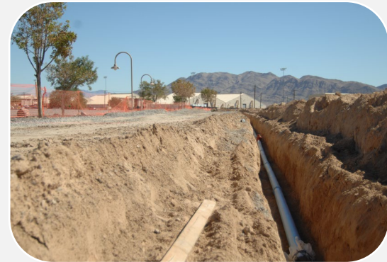
Shocking Distribution Repairs/New Construction
