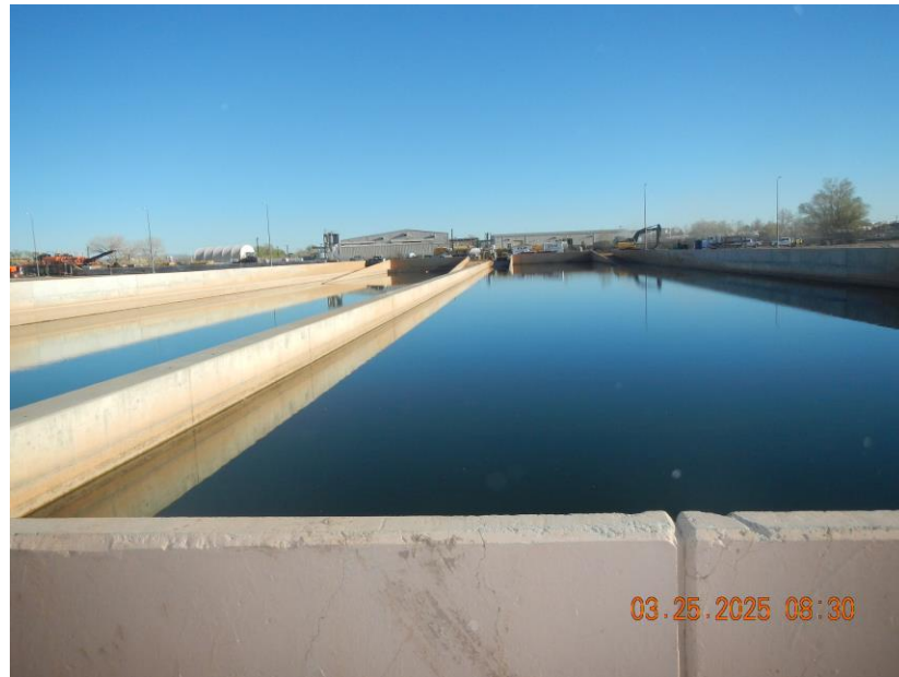
Albuquerque Water System Pre-sedimentation basin
