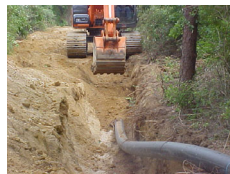
HDPE pipe installation
