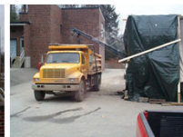
Hauling Solids Away
