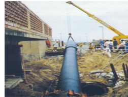
HDPE pipe sliplining job shown
