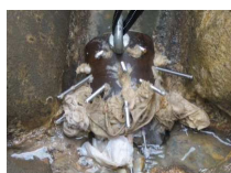
Porcupines are used to scour pipe walls of hardened debris, roots, & grease
