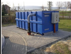
Left: Biofilters can treat odors in air vented from sewer
