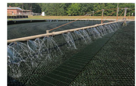
Trickling Filter
