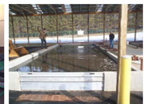
Gravity Filter Bed
