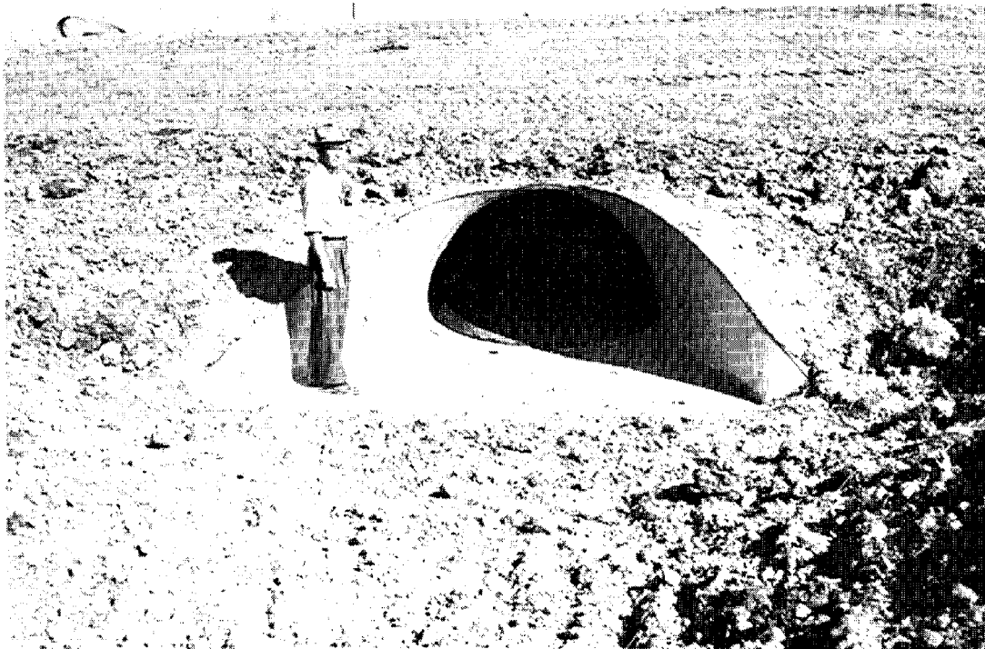
Prefabricated entrance section on pipe drop
