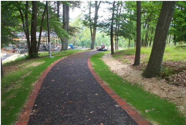
Porous asphalt path at Gray Towers Natl. Historic Site, PA
