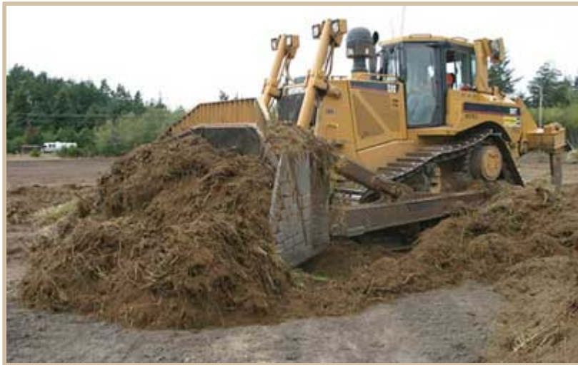
A native topsoil being spread back over a restored site. Photo: Dave Ledig, U.S. Fish and Wildlife Service
