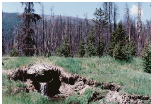
Figure 57–Drainage patterns changed when a road was built across this meadow. The water can drain through only a few culverts, which concentrates the outflow and causes down cutting that has led to an incised stream.
