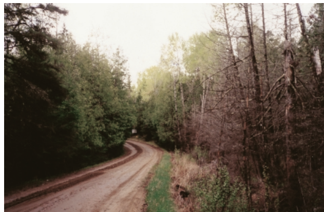
Figure 56–Cedars are very sensitive to hydrological changes. The cedars (at right foreground) died because of the road construction and because the subsequent compaction and settling of the roadbed changed the hydrologic regime. The water became impounded around the cedars and they drowned. Their deaths further impacted cedar regeneration because increased deer browsing makes regeneration difficult, if not impossible.
