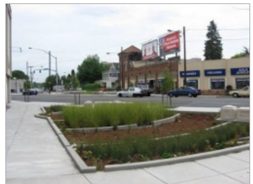
Bioretention can be used to create a green street by managing street and sidewalk runoff (Source: Abby Hall, US EPA)
