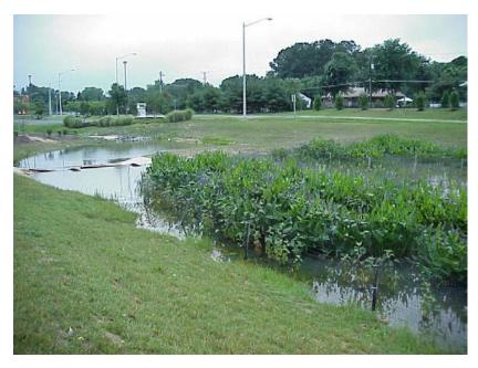
Constructed Stormwater Wetland. Note vegetation protected from waterfowl by netting system.
