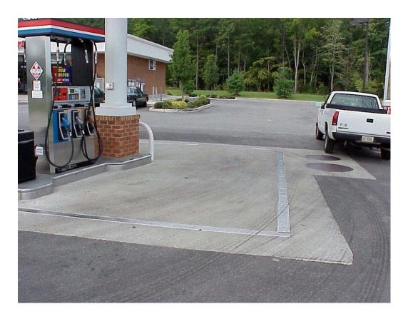
Manufactured BMP Systems. Manufactured systems can be selected to address specific pollutant sources. This trench drain surrounds fuel handling area of a service station to direct any spills or other identified petroleum based contaminants to a manufactured system designed specifically for fuel or hydrocarbon containment. Note: fuel area is under cover which serves to limit the design flow entering the system.
