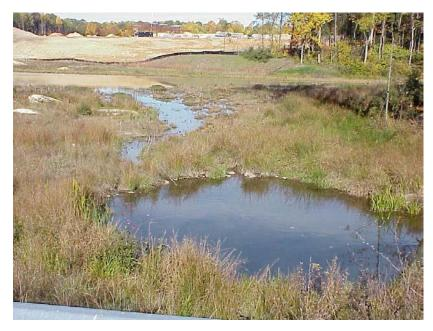
Forebay and Constructed Stormwater Wetland incorporated into regional retention basin design.
